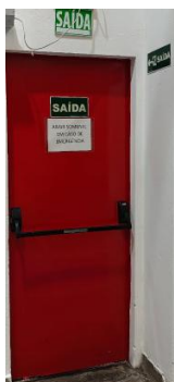
Photo 21 Emergency exit door.jpg
