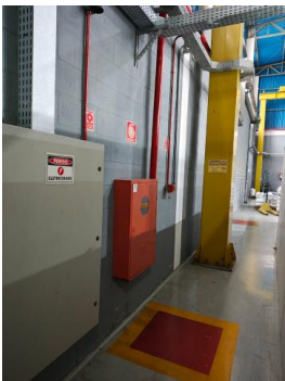
Photo 17 Electrical board and Waterhos-Hydrant .jpg
